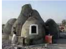
Private residence built in Bam, Iran after the 2005 earthquake
