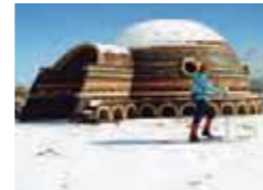
Hesperia Lake RUMI Dome was built as part of a Museum and Nature Center project
