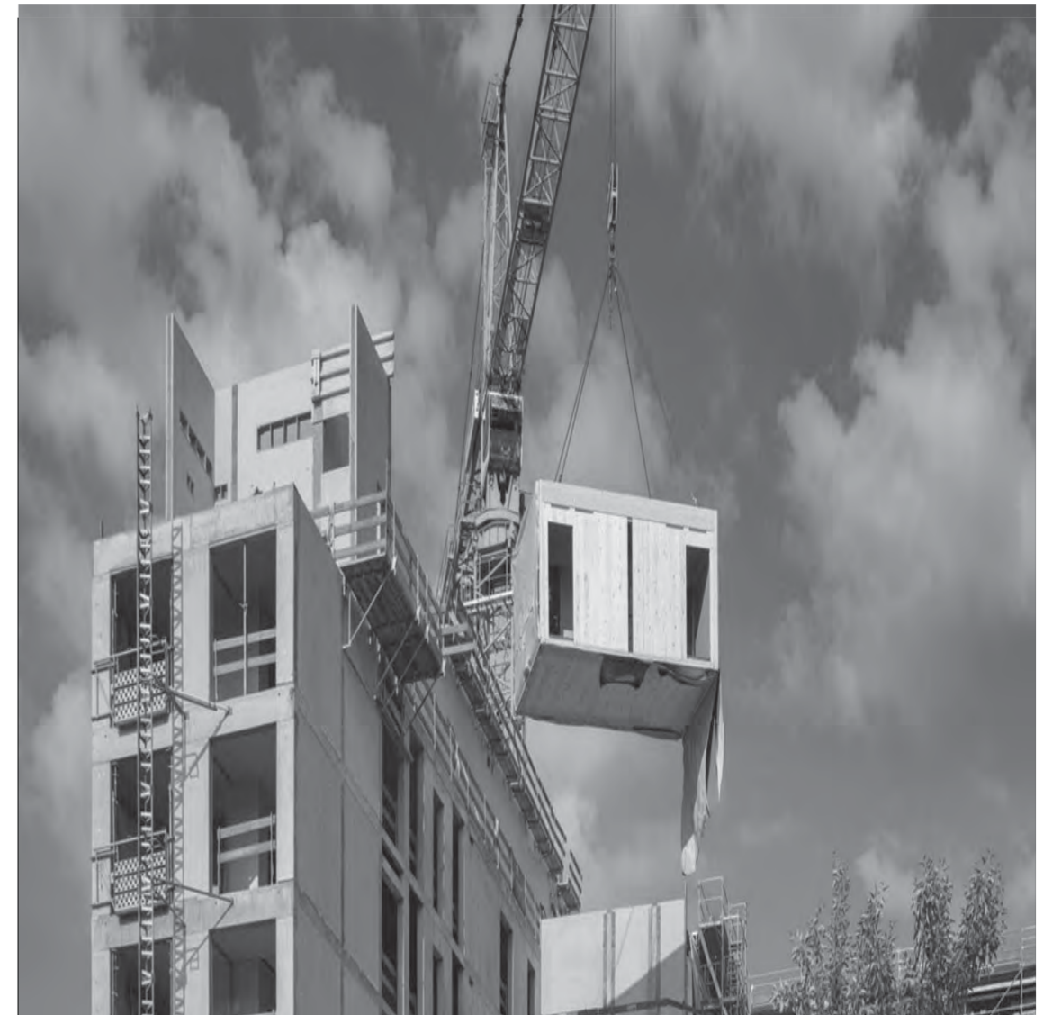
Fig.3 "Modular Building" HVP Magazine, 18 February, 2022
